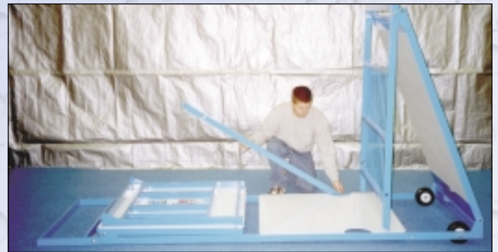
Prop as shown and attached angle braces. Raise roof, attach to angle braces.
